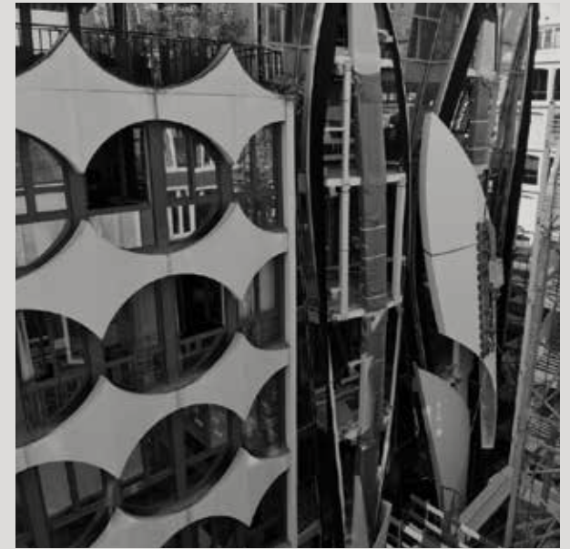
Installation of petals
