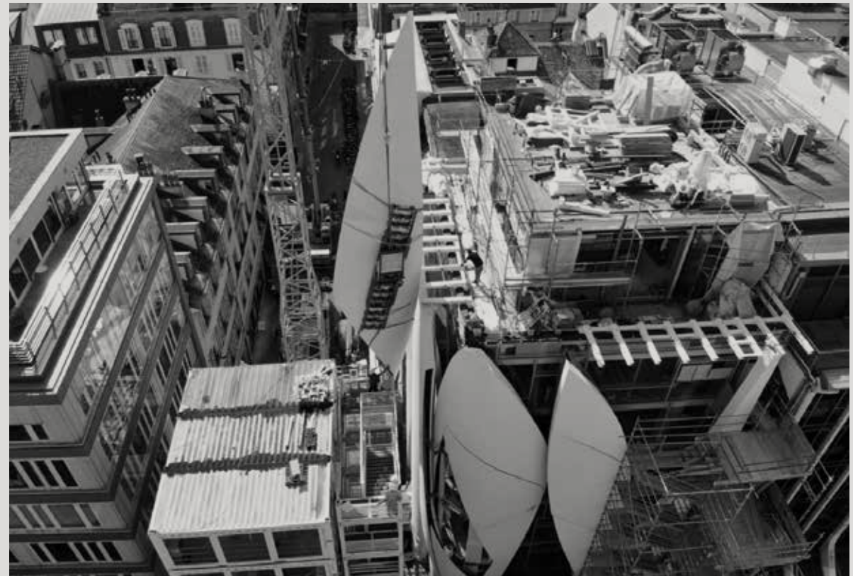
Lifting of GFRP modules
