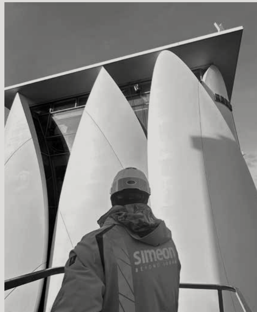
Supervision of petals installation
